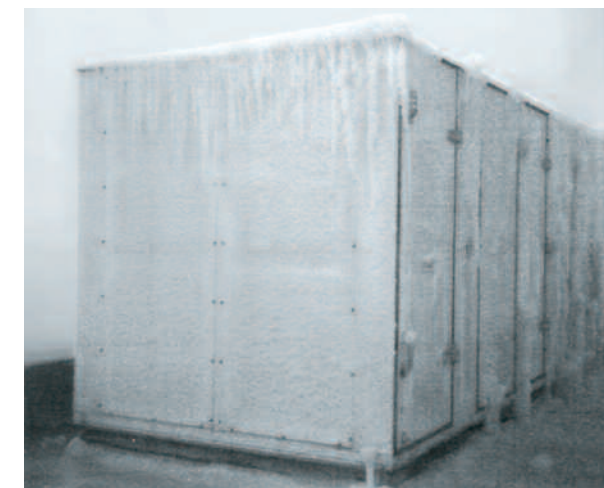
Conditions do not always have to be 'extreme' for extreme problems to arise. These images of totally ice-bound air intakes were taken in northern Germany in ambient conditions of around 0 °C.
